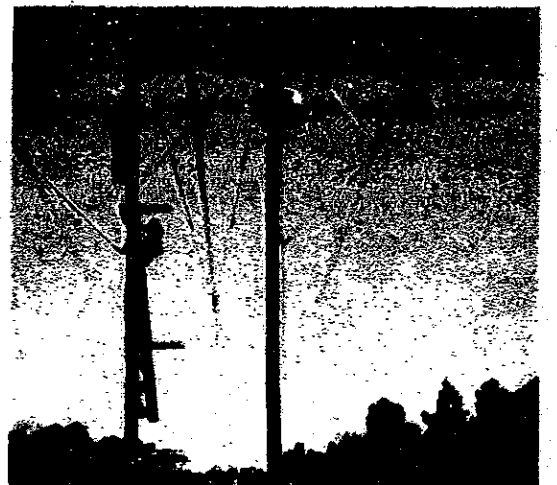
The old structure has been dismantled, and new poles have been set. Here, they are installing the cross-arm with insulators already attached.
