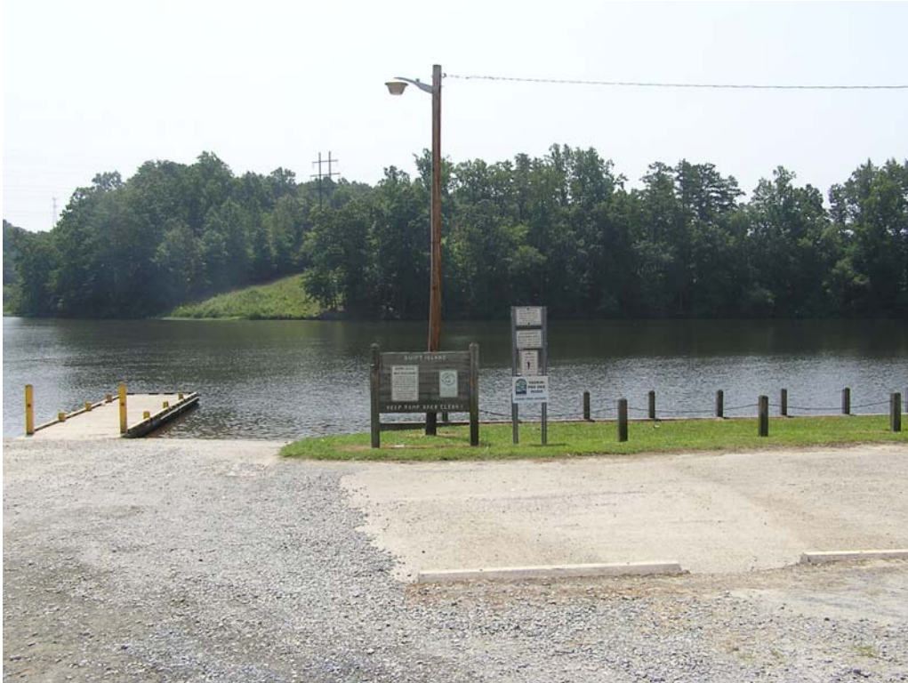
Swift Island public access boat launch site.
