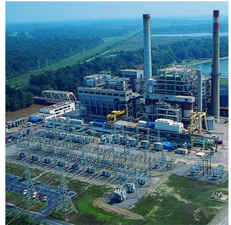
397-MW H.F. Lee coal plant in Wayne County, NC
