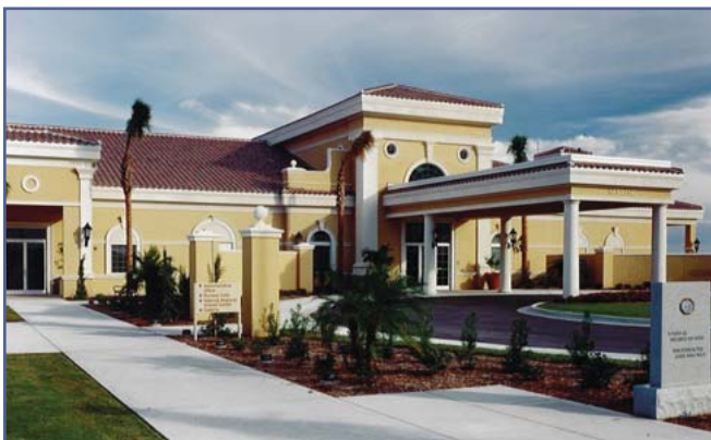
Sebring Regional Airport Terminal Building. The airport and its commerce park generate an economic impact of well over $200 million annually.
